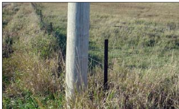
Above: Fencing this close to a power pole can be dangerous for linemen as they climb the pole to make repairs.
