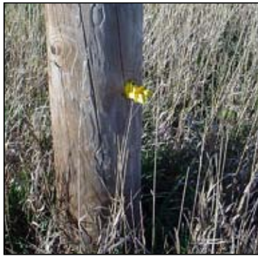
Safety codes also dictate that you cannot attach your own wiring system to Western's poles. Including electric fence wire shown above.
