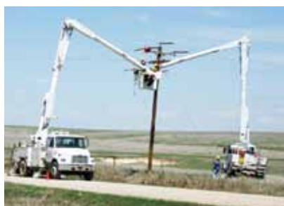
Western's crews and contractors will straighten 7,000 existing poles.
