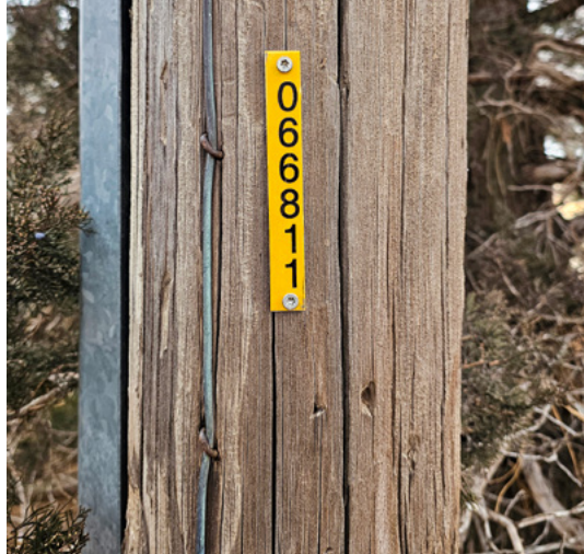
Every pole on Western's electrical system now features a unique identification number that directly corresponds with the cooperative's mapping and operational systems.
