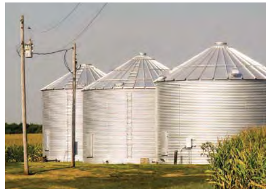
Building a structure too close to overhead power lines can create an electric shock danger during and after construction.
